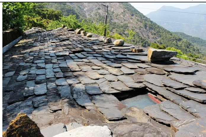
仿百步蛇鱗片層層堆疊的石板屋頂
